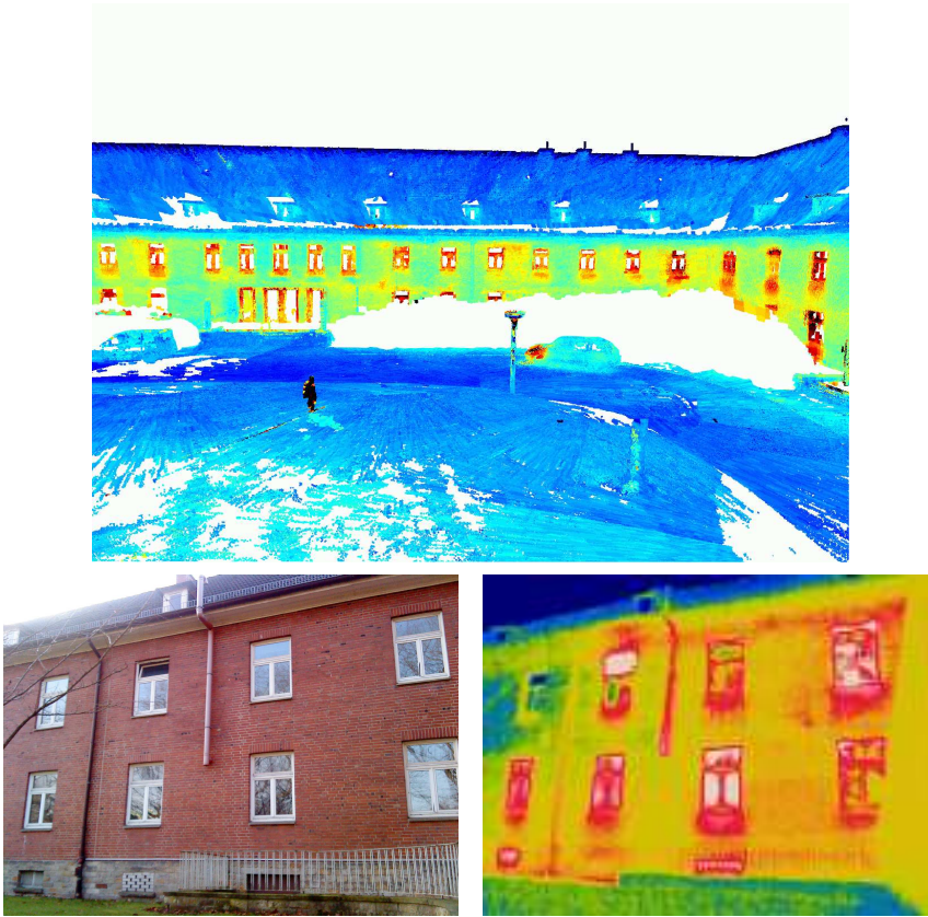
Fig. 2: Above: The campus center of the Jacobs University as a 3D point cloud with thermal information and filtered vegetation [Elseberg et al(2011)]. Below: Photo of eight windows (left) and the corresponding infrared image (right). In the thermal image heat losses are clearly detectable. In the top row the windows show different temperature distributions. The first window on the left belongs to an empty office which is not heated. The top part of the second window is open. The third window is closed and has proper insulation. The fourth window shows unusually high temperatures. This was caused by a partially detached rubber insulation strip that allowed the air to flow through.
